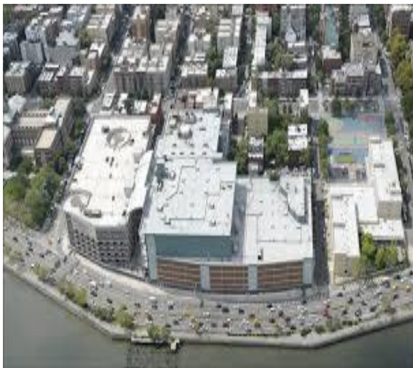
Existing East River Plaza Shopping Structure
